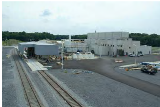
Figure 3.2. DUF 6 Facility Construction Activities
